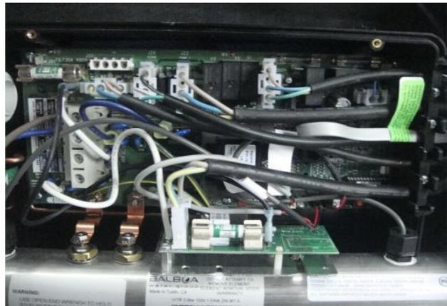
**Step 3:** Then connect your home power supply to Live Wire and Neutral Wire location on the control box.
