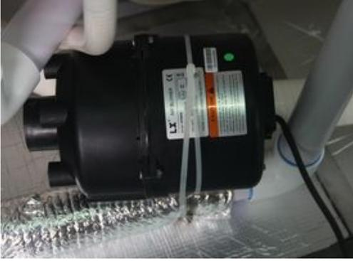
**Step 3:** Then install the blower in where it should be installed with screws by necessary tools.
